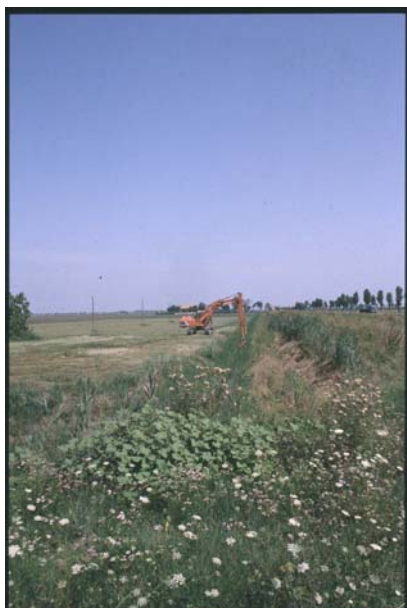
Figure 2. Digger carrying out excavation work in a ditch.
